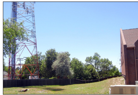
Figure 5. The TV and cellular transmission tower, left, is only 90 feet from the Fire Station No. 1 structure, right, and lightning energy from the tower could have passed to the station through the ground before repairs were
