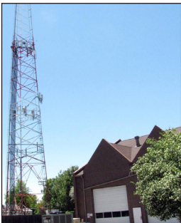
Figure 4. A privately owned, 200-ft transmission tower stands on the property immediately adjacent to Fire Station No. 1. The fire station does not utilize the tower; however direct lightning strikes to the tower or induced currents in the tower during storms did affect low-voltage electrical systems in the station.
