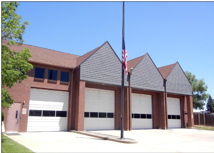
Figure 1. The Cunningham Fire Protection District's Fire Station No. 1 also houses administrative headquarters. From 1985, when the district bought the building, until 1999, electrical disturbances driven by summer thunderstorms caused increasingly expensive and hazardous and potentially fatal damage to communications systems.
