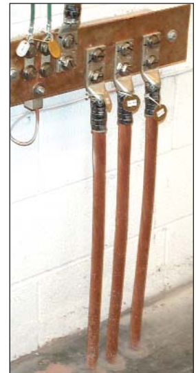
Figure 7. Penetrations through floors are lined with PVC to avoid the risk of fire. Metallic penetrations can suffer hazardous resistive heating when large surge currents pass through the grounding conductors. Connection lugs are tinned copper.
