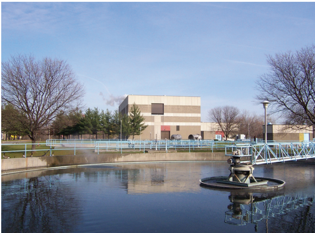
The Menands, New York, treatment plant operated by the Albany County Sewer District was one of two facilities selected by NYSERDA to evaluate ultra-high efficiency, copper-rotor motors. As in other industrial settings, motors account for much of the plant's electrical energy consumption. Photo: Albany County Sewage District
