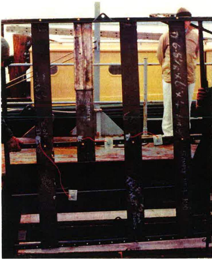
Figure 15. Raft Site. Mounted panels being lowered into place.
