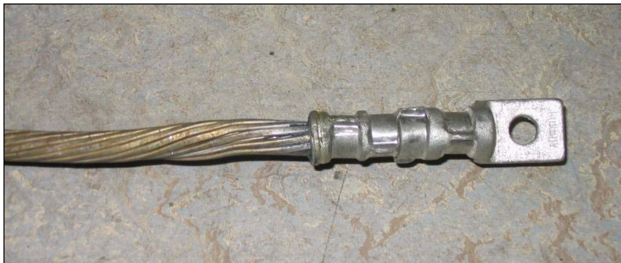
Figure 10. Typical remade equalizer using a new compression connector.
