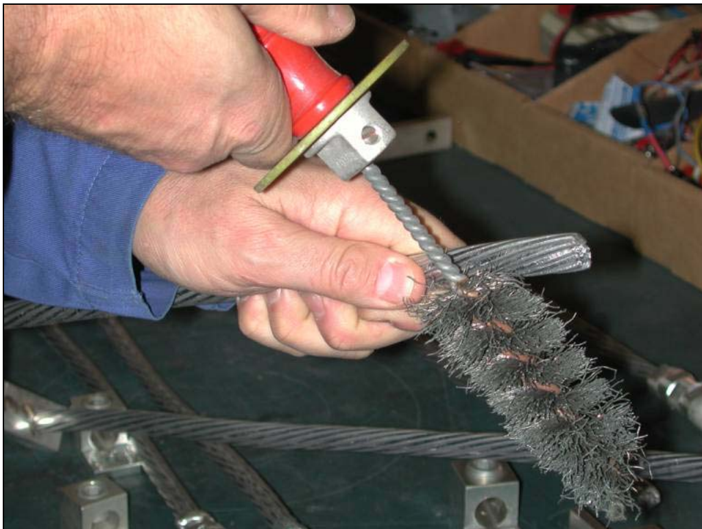
Figure 2. Wire brushing conductor samples during installation.
