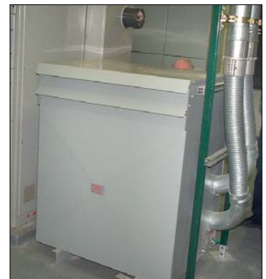
Figure 3. A 300-kVA transformer located on the building's 27th floor supplies 3-phase 208Y/120-V low-voltage service to floors 17 through 27. Poorly made high-resistance connections to the transformer caused large current differences on parallel conductors leading from the transformer. Loose connections on aluminum feeder cable throughout the system caused the transformer to overheat.
