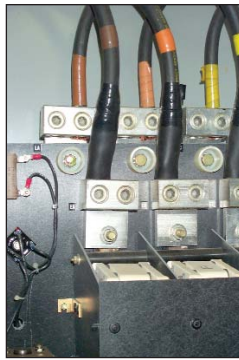
Figure 9. New, correctly installed copper feeder connections inside a breaker panel. Note that connections are now properly bonded at tinned-copper connector bars. Compare this installation with the cables shown in Figure 5 .
