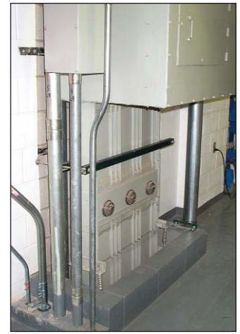
Figure 2. A 1,350-A/480-V copper bus duct leading from the Capitol Square basement to the building's utility loft on the 27th floor, from where it feeds the 300-kVA transformer that supplies 208Y/120-V service to the 17th through 27th floors. Aluminum feeder cables had loose connections, which contributed to the voltage drop experienced on the upper floors.
