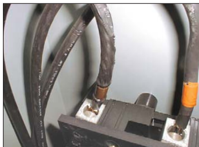
Figure 10. Evidence of overheating is seen in the damaged insulation on this aluminum conductor leading to the chiller disconnect switch on the building's 27th floor. The aluminum has been replaced with copper of the same wire gage.
