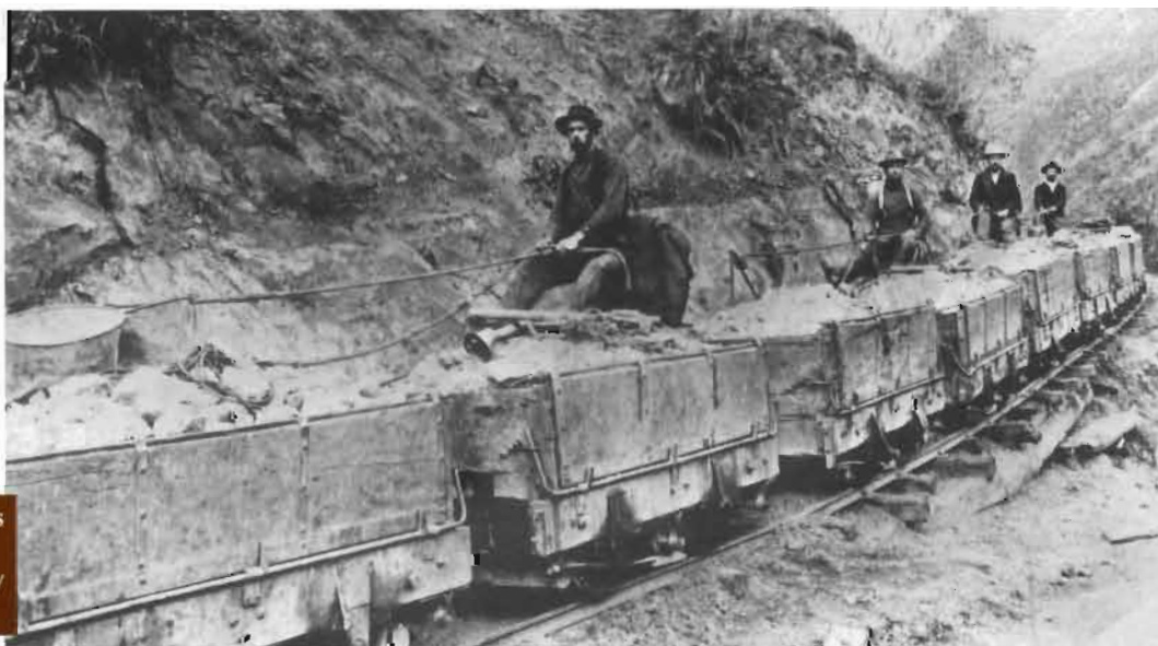
Figure 1 - In 1882, ore cars rumbled down the canyon from the mine propelled by gravity.
