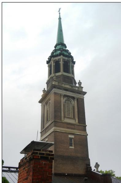
*Figure 8. St. James's 160-ft, copper-clad steeple stands at the front of the church. Although a 1994 lightning strike probably hit the steeple, destroying the church, the steeple itself remained relatively unharmed. The steeple was not grounded before the lightning strike. Now, the steeple, the periphery of the church's roof and all rooftop equipment are protected by strike termination devices (Franklin terminals), all bonded to a securely grounded, 100% copper lightning protection system.*
