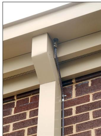
**Figure 7.** Rather than looping down-conductors over gutters, Loehr Lightning Protection Company routes them through the overhang when necessary, sealing the penetration with a solid copper rod enclosed in a water-tight fitting. The result is a cleaner, less conspicuous installation.
