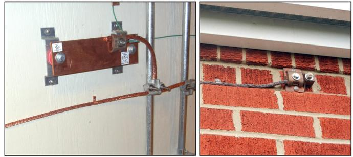
**Figure 6.** Indoor grounding bus with wall penetration (left); the right-hand photo shows one of several outdoor wall penetrations, from which the heavy-gauge copper conductor to the left of the penetration lug leads downward to a driven earthing electrode.
