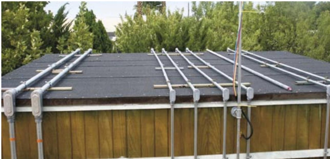
**Figure 4. Conduits passing over roof of commercial building**
