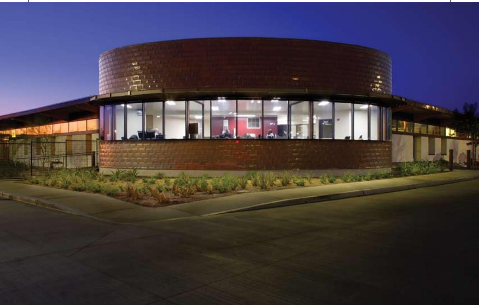
acts as trim on the building's 8-foot (2.4-m) roof overhangs, which block unwanted heat and ultraviolet rays from reaching the building's interior in the hot summer months and keep the walls dry during rain storms. The administration building's interior courtyard also features the copper shingles.
