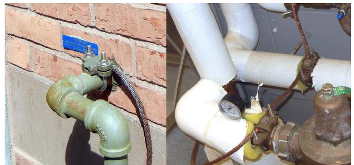
**Figure 3.** Braided lightning conductor (29 strands of bare 17-gauge copper) is shown bonded to the fire station's water supply line, left. Note the use of UL96-approved copper alloy mechanical clamps. The clamps resist loosening and corrosion. Similar connections were applied inside the building.
