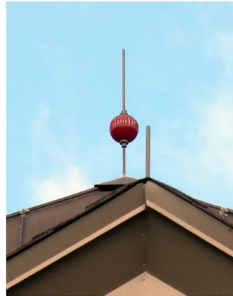
**Figure 1.** Air terminals (strike termination devices) are mounted at a code-mandated maximum 20-ft interval on the roof of the Simsbury Main Station No. 1. The decorative terminal is one of several installed for architectural reasons. Note the braided copper lightning conductors mounted along gable edges.
