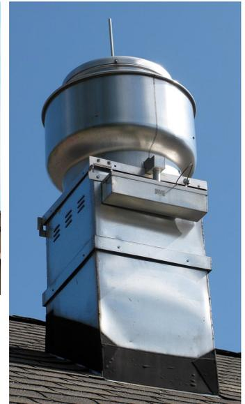
**Figure 2.** Rooftop ventilator with air-terminal. The otherwise ungrounded ventilator is within a six-foot strike distance of the lightning protection system's cabling (not shown) and is therefore connected to it.
