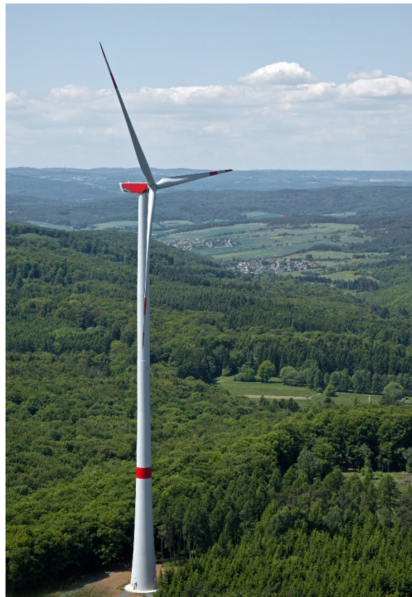
Taller towers require more copper cable. Example of a Nordex 2.4 MW wind turbine with 117-meter rotor mounted on a concrete and steel 141-meter hybrid tower (source: Nordex)
